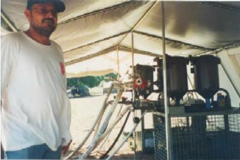
The Austrian army took over the water purification
